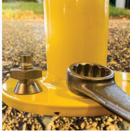
Breakaway Nut Pre Installation
